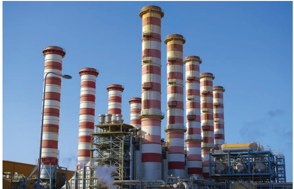
❖❖❖ Ras Abu Fontas: one of Qatar's largest power and desalination plants
