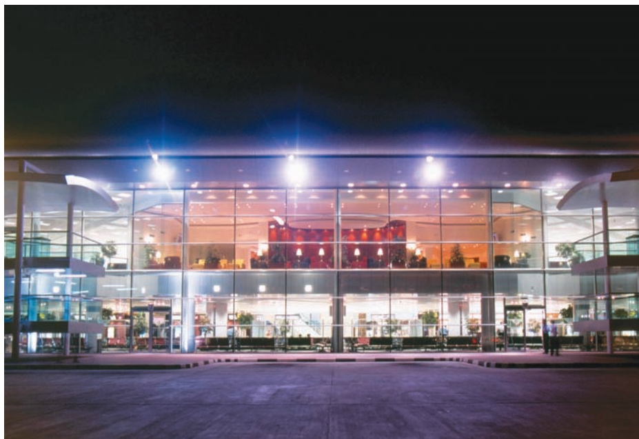
NDIA: one of Qatar's largest and most impressive infrastructure projects
